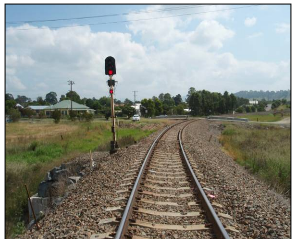
Figure 1: Outer home signal and Phillips Street level crossing.
