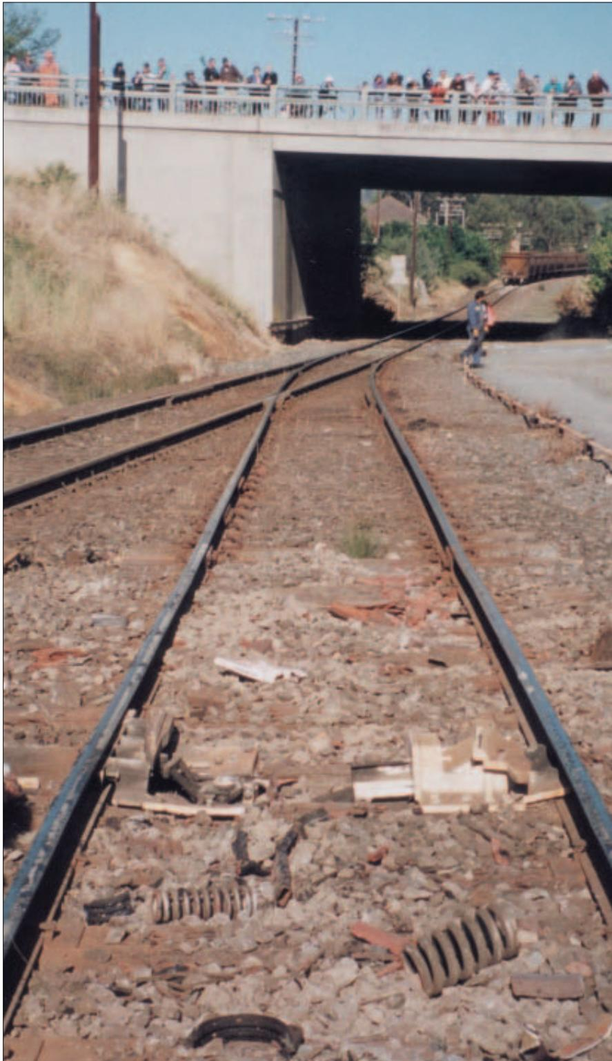
The points at Ararat were interlocked with the derailer on the No. 2 Road but were not interlocked in any way with signals or the Safeworking system on the main line, nor were they provided with point indicators to warn Drivers on the main line that the points were not set for the main line.
