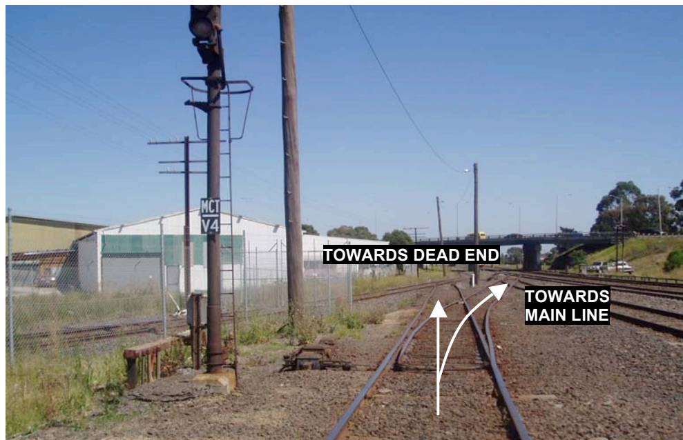
Figure 14: 'Natural trap' cross-over style protection at McIntyre Loop
