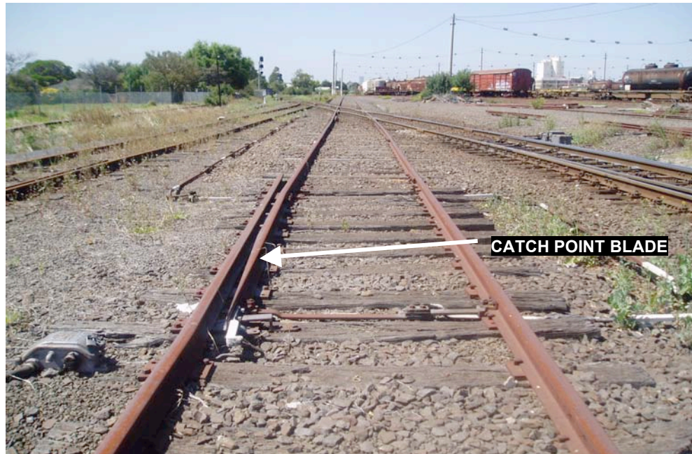
Figure 12: Catch point fitted with throw off rail and wheel ramp at Sydney Central
