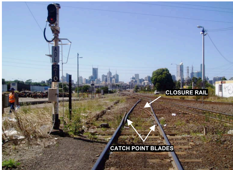
Figure 13: Double blade catch-points at South Dynon
