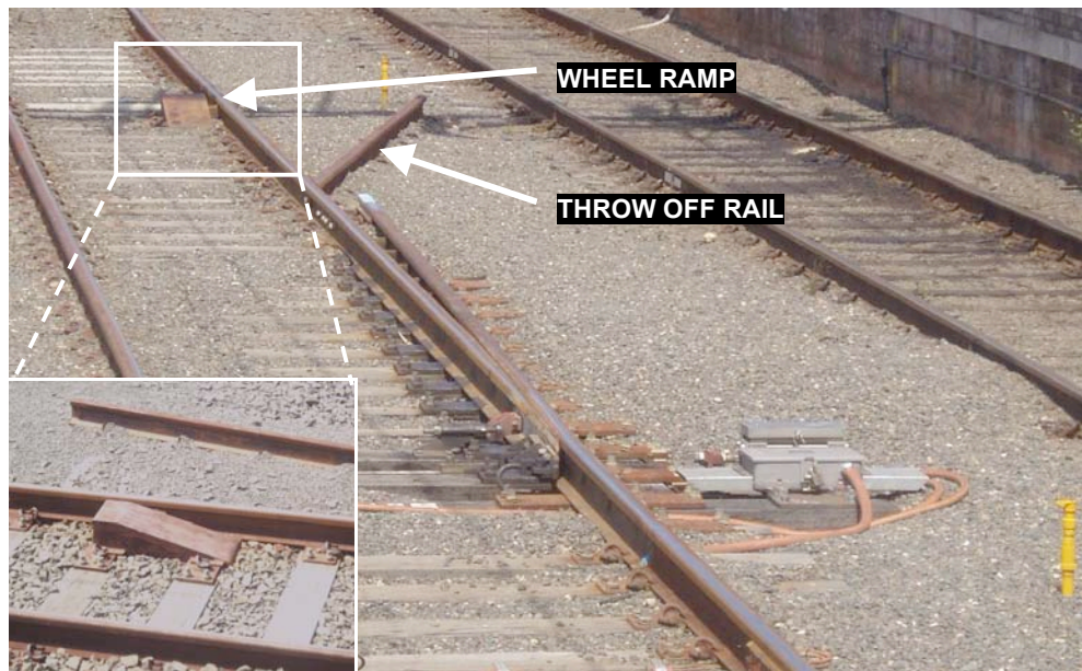
Figure 12: Catch point fitted with throw off rail and wheel ramp at Sydney Central
