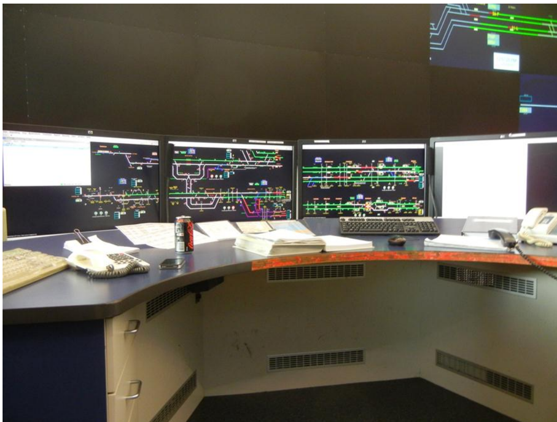
Figure 5: Sydenham signal complex – Meeks Rd-Campsie control panel
