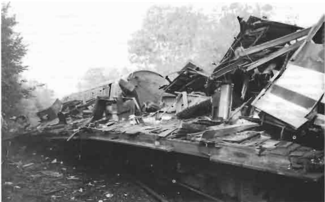
The frame of the leading coach of the Up train showing the destruction of the superstructure
