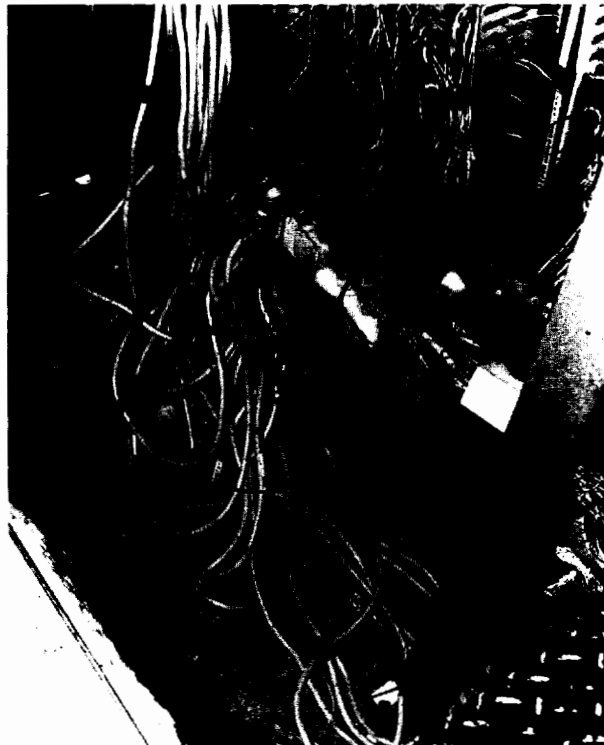
Damaged wiring, Motherwell Signalling Centre
