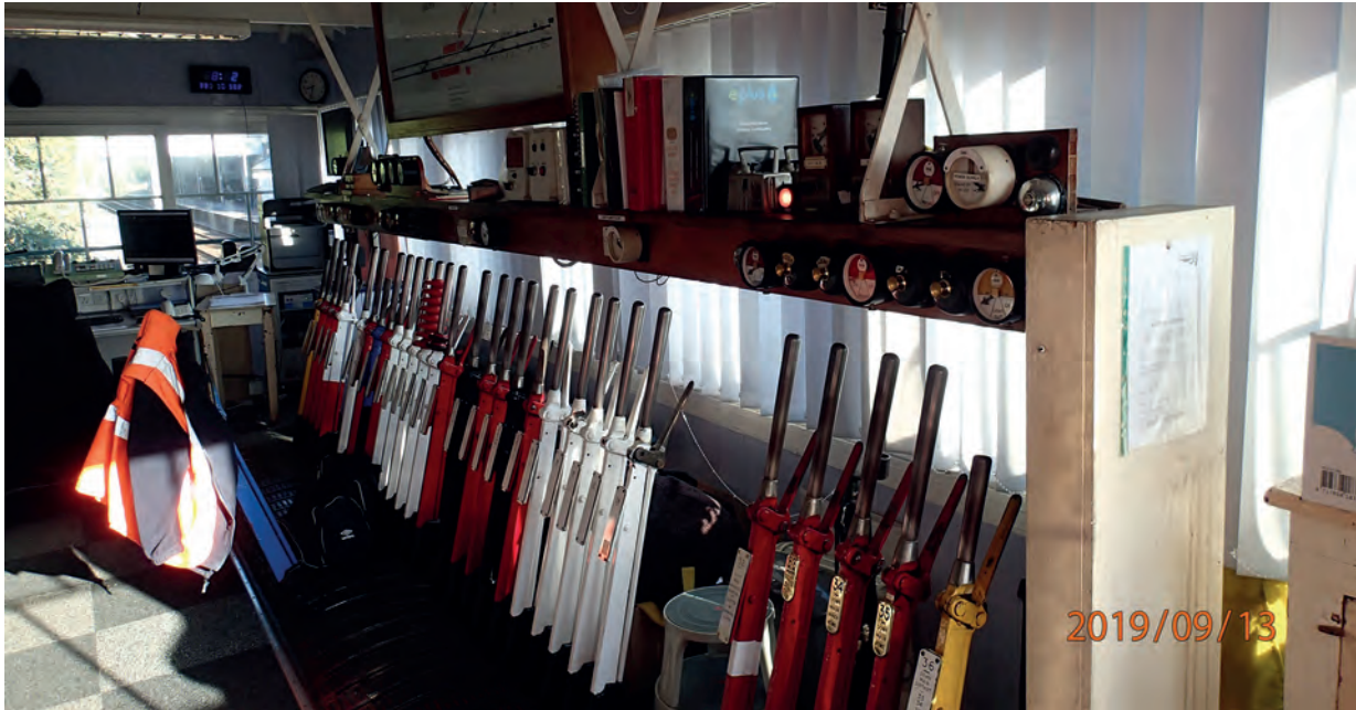
Figure 1: Example of a lever frame signal box
