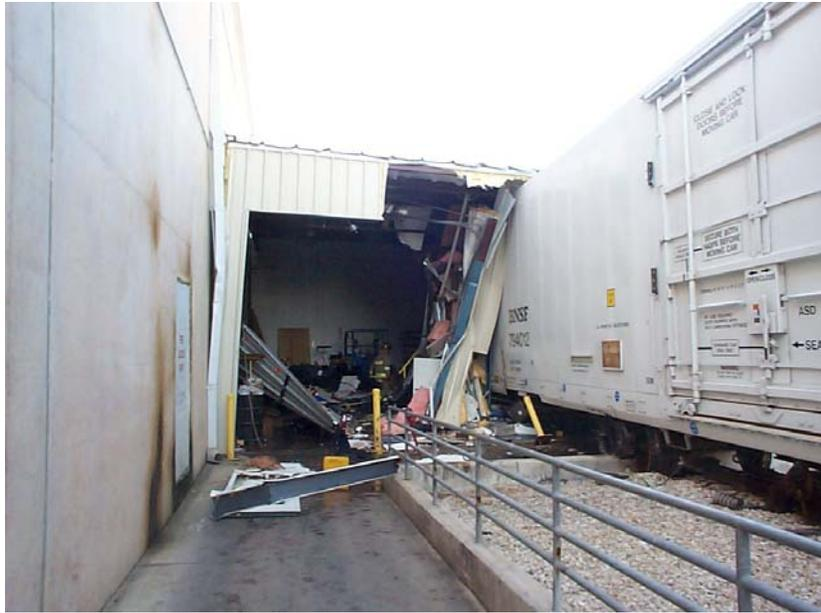
**Figure 1.** Damage to Crystal Cold Storage maintenance building.
