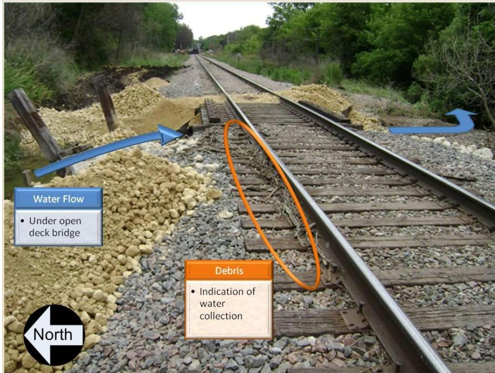
**Figure 5.** Photo shows storm water debris on the track, near the open deck bridge (0.1 mile west of the accident site). Water flow under open deck bridge is also indicated as flowing in southeast direction.
