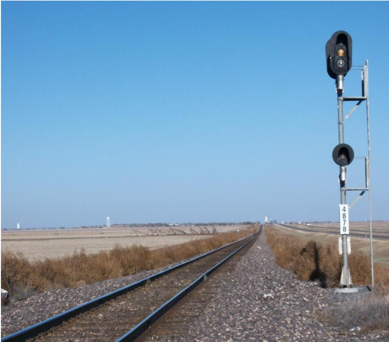
**Figure 3.** Typical signal light on UP Pratt subdivision.
