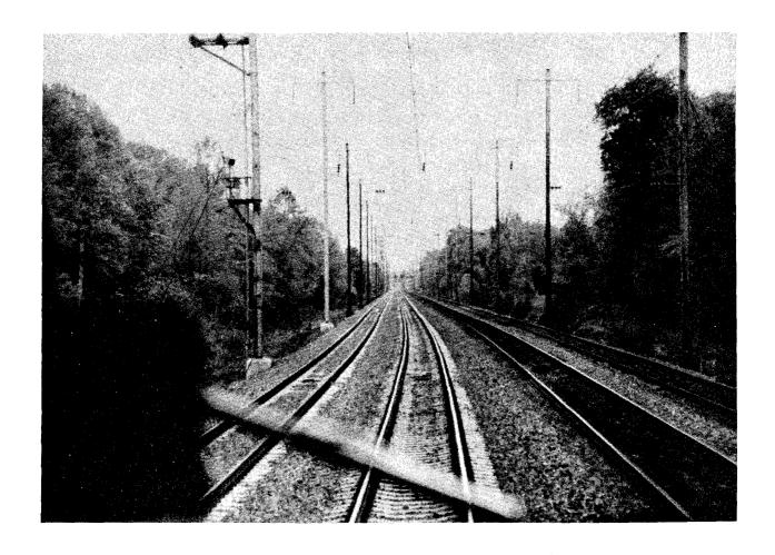
Figure 10. Code chande point CS-806 as seen from a northbound train on track 2. The nearest catenary support poles mark the location of the code change point. The Gunpow home signals are in the distance.
