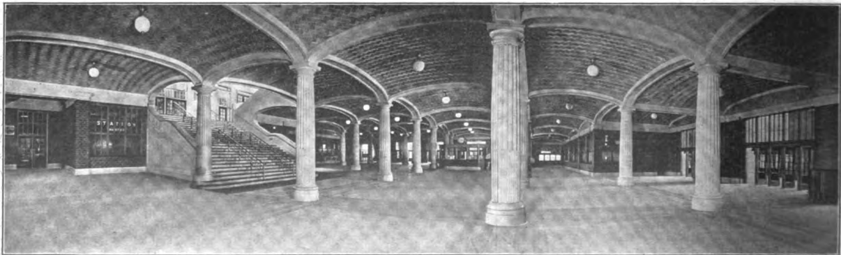
Public Court on Ground Floor.
