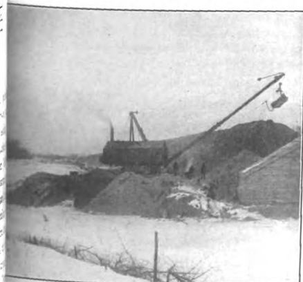
The Excavator Making Long Fill from Adjacent Borrow Pit; Milwaukee, Sparta & Northwestern.
