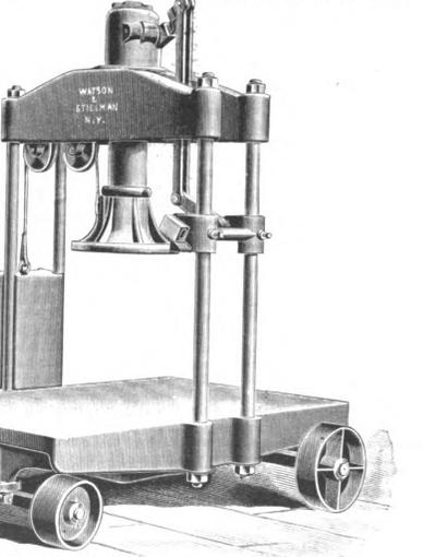
according to the proposed standard drop tests of couplers given in the M. C. B. Committee's report. The apparatus consisted of a 1,640-lb. drop mounted in a suitable vertical frame and raised by a hoisting engine. The foundation consisted of 5 ft. of masonry, 5 in. of timber, bolted together to form one solid floor, and 8 in. of cast iron in a block weighing 2,600 lbs. The tests were
