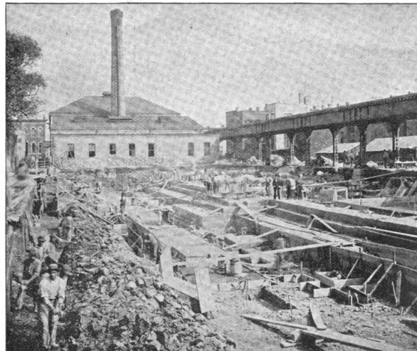
Fig. 5.—Foundations of Power House, West Side Metropolitan Elevated.
