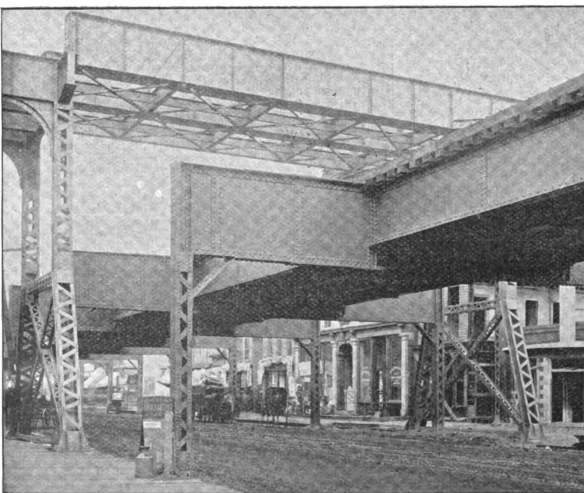
Fig. 3.—Crossing of Milwaukee Avenue branch of West Side Metropolitan Elevated over the Lake Street Elevated on Lake Street.
