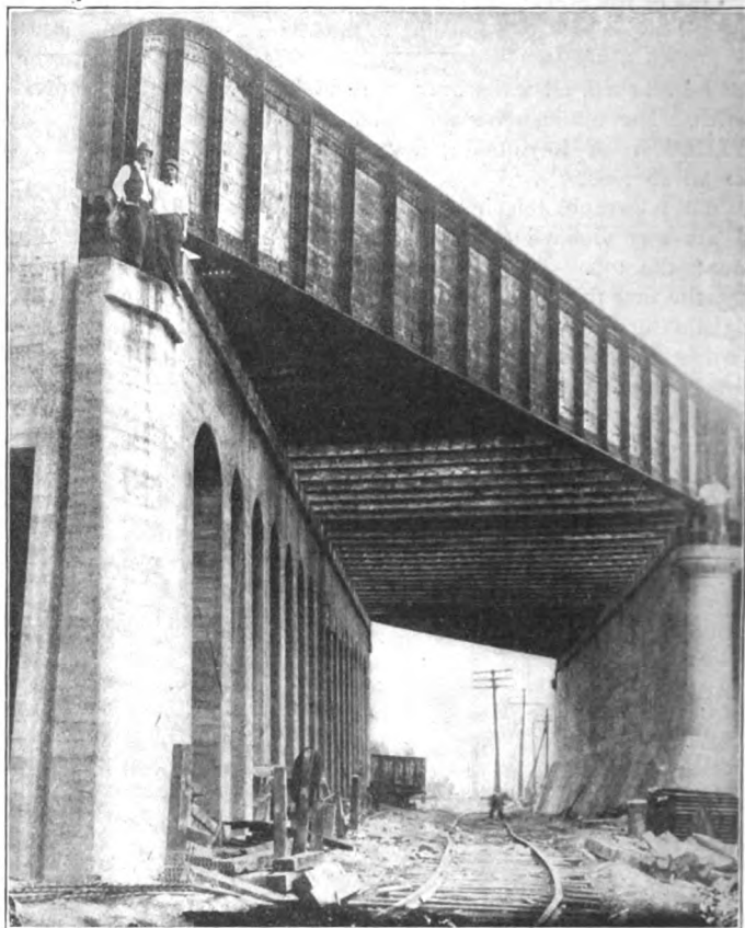
One Span of the Seventy-Ninth Street Structure Showing Main Girders, Floor System, One Abutment and One Pier Before Concrete Encasements Were Placed
