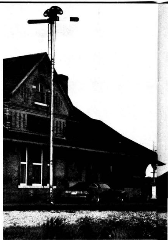
OPERATOR at West Liberty, Ia., "copied three west" (above) for 57's train, the Extra 351 West, which picked them up at speed from the order stand (right). To ease dispatchers' load, Rock had several local-control CTC installations like this.
