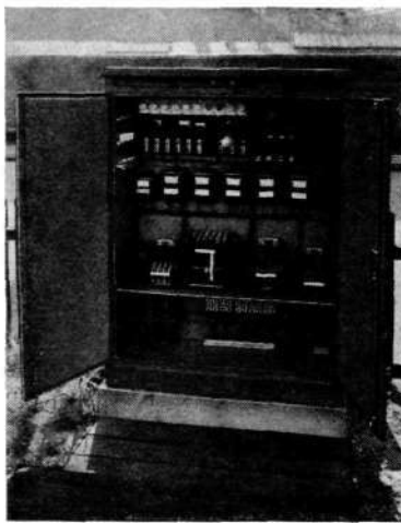
Fig. 5 Relay cubicle
