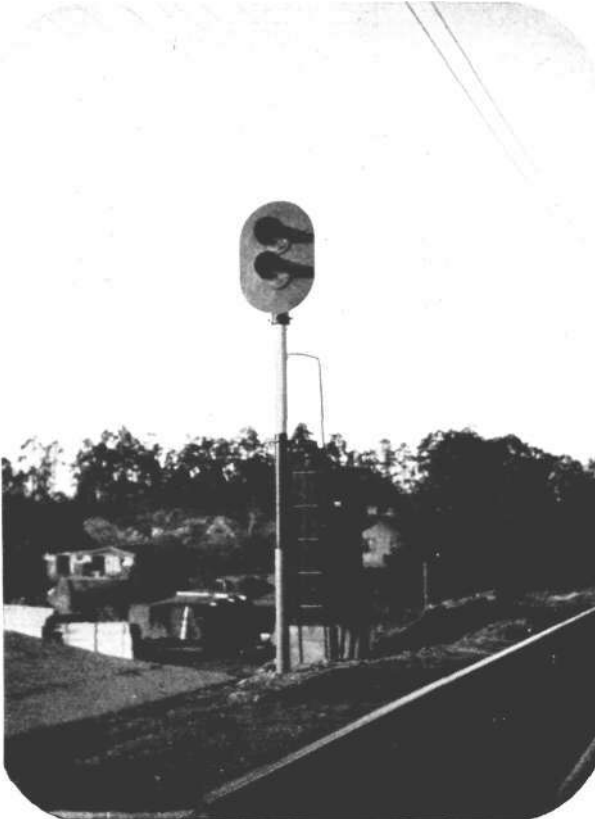
R 681 Fig. 4. Light Signal and Relay Cabinet.
