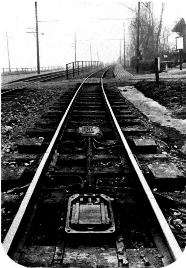
Fig. 8. Impedance Bond.
