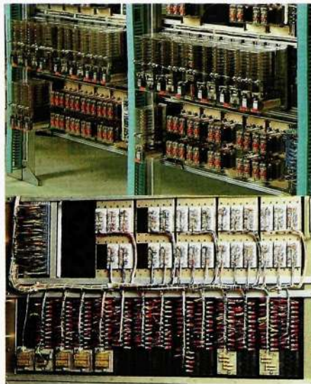
Fig. 1 The degree of safety obtained with robust relays, large insulation distances between the circuit elements, guided contacts and simple circuit structure corresponds to what is obtained with large information and system redundancy in a computer controlled system
