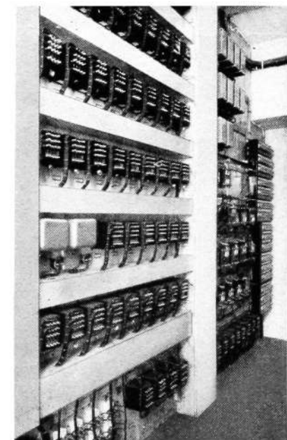
Fig. 5 X 4625 Interior of the relay room where JRG relays, transformers and fuses are mounted on a wall
