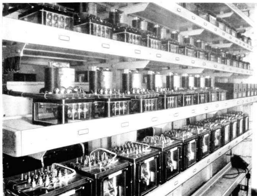
Fig. 4 X 6404 Interior of the relay room Most of the relays are set up on wooden shelves.
