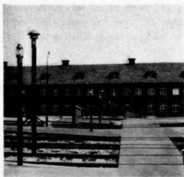
Fig. 7 Light signals and bells for protection of level crossing
