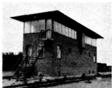
Fig. 11 Cabin II (Master Cabin)
