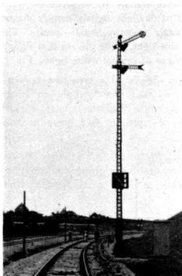
Fig. 5 Entrance signal with direction indicator
