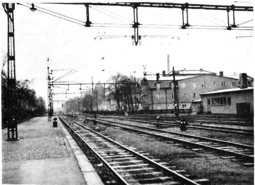
Fig. 1 Dwarf signals in the station track area
