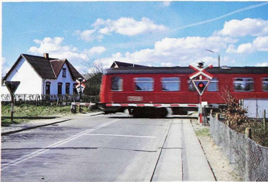
Fig. 10 Control of 66 level crossing plants on the line is integrated in the interlocking functions
