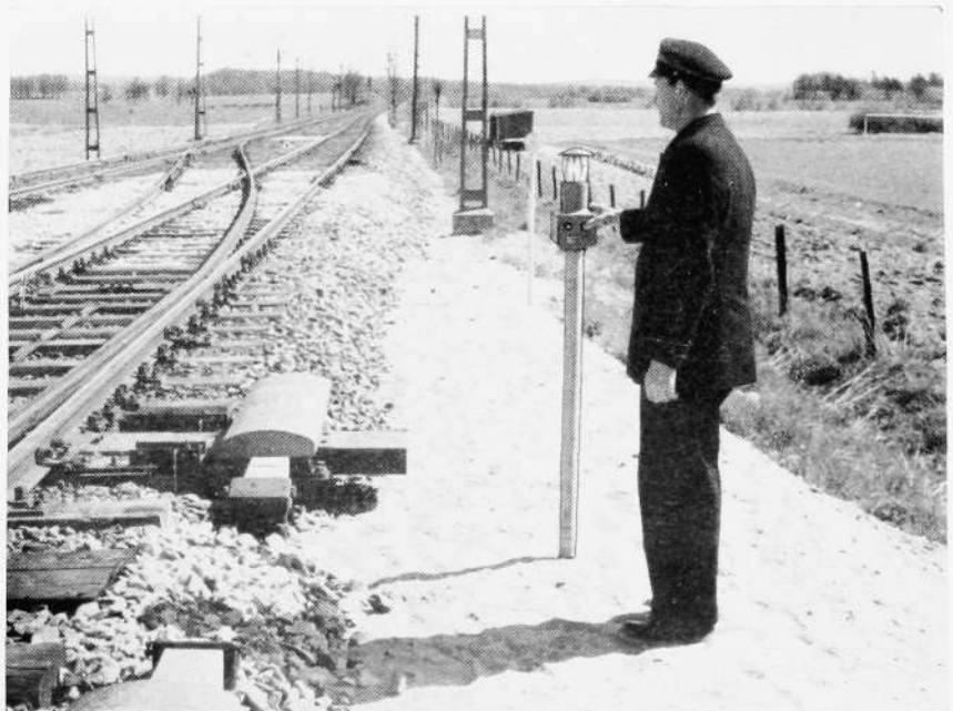
Fig. 5 X 6607 Local lever at the point. The lever contains a lower part with push buttons and on top a lantern fitting with drum lens. A yellow light in the lantern indicates that local point operation is permissible.
