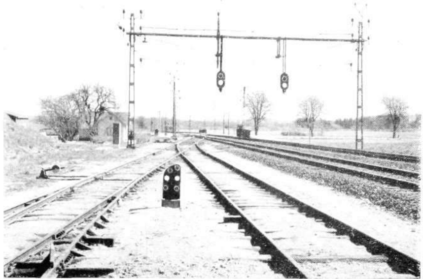
Fig. 8 X 6610 Colour light signals for exit from the two tracks. A dwarf signal is used for the side track with six apertures of which the two bottom lights are green.
