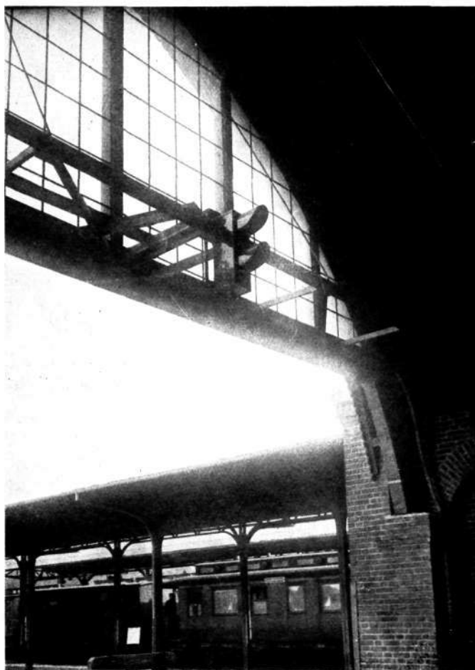
Fig. 4. Repeating Signals on Gable of Train Shed.
