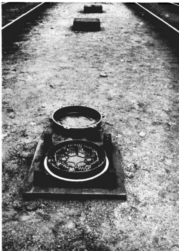
Fig. 8. Cable Distribution Box.
