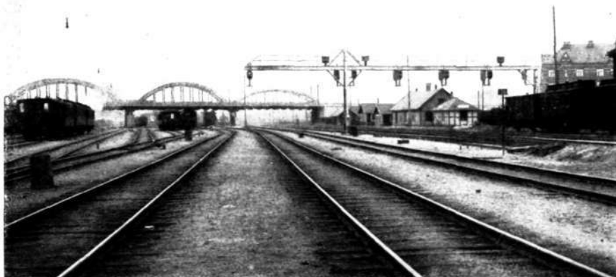
Signal Bridge, looking away from Track Yard.
