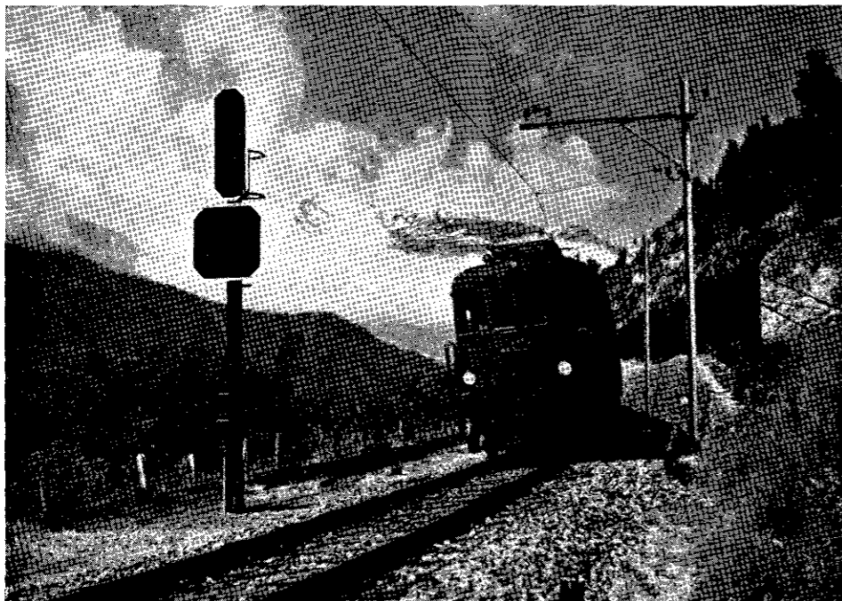
Fig. 1 Home signal, with inner distant signal below, on Lötschberg line
