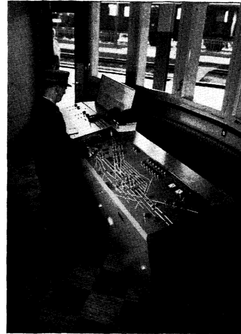
Fig. 6 Supervisor's control apparatus at Zug, with buttons for sending releases to signal boxes
