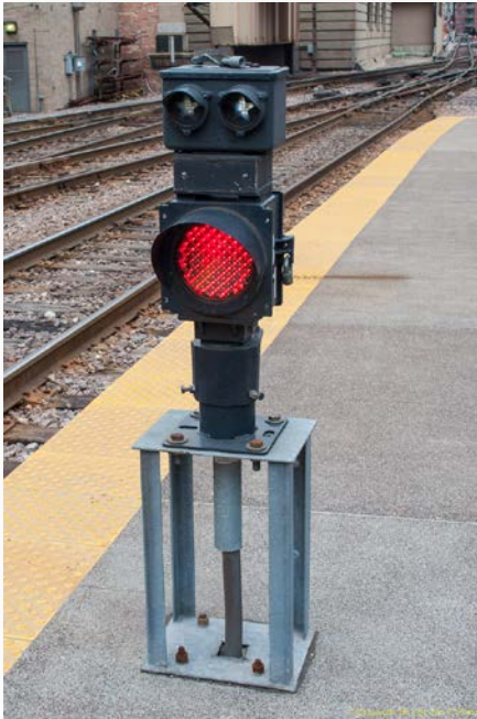
Here's a modern-day view of signal 131, facing north toward the station throat. Signal 131 governs outbound moves from station track 3.
