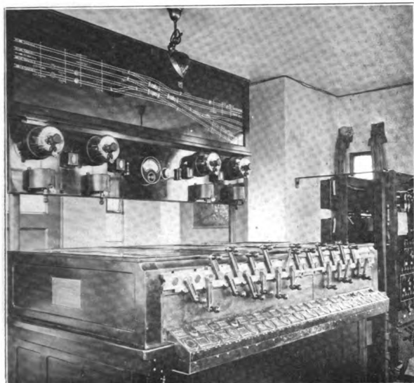
Fig. 30. Interior of Operating Room, Columbus Avenue Tower.
