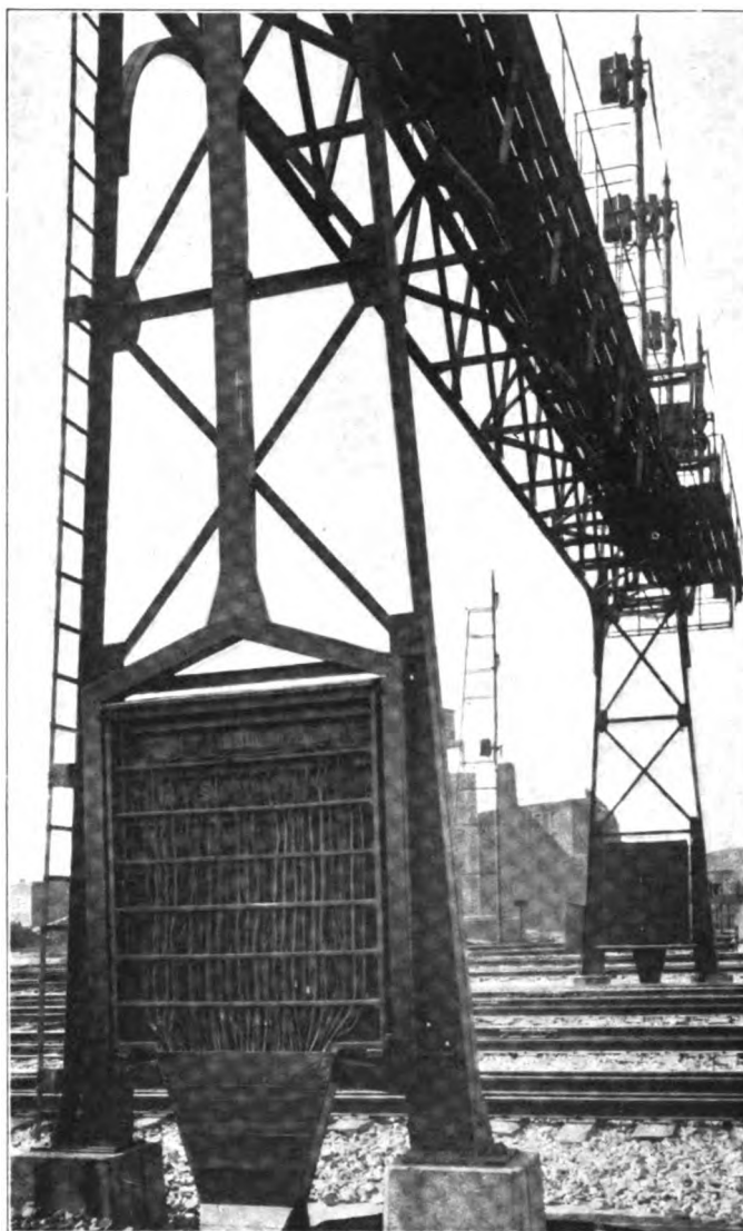
Fig. 9. Rear of Relay Box with Back Removed, Showing Arrangement of Wires and Cables.
