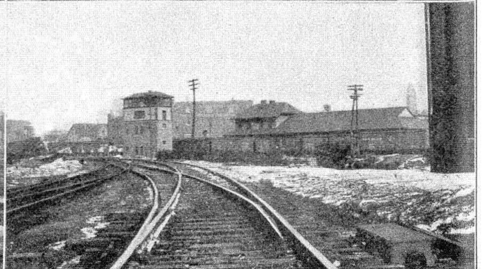
A Hayes Derail Layout A Single Switch Layout
