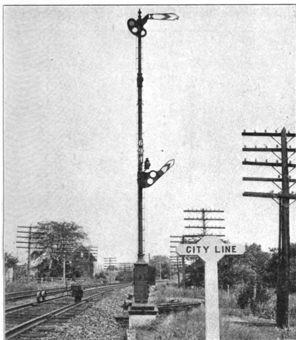
Fig. 1—B. & O.—Automatic Signal with Auxiliary Arm
