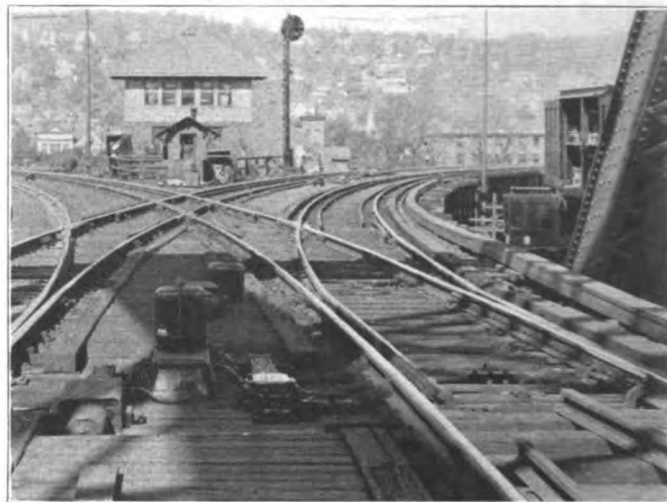
An Assembly of Electro-Pneumatic Switch Movements and Valves
