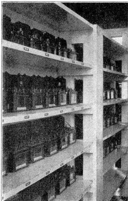
Relay Rack on First Floor of Tower, Note Absence of Wires
