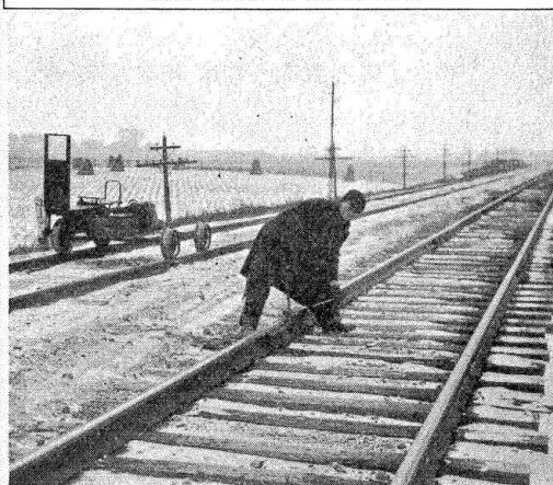
Above—The bonding is the same type on both A-C. and D-C. sections, using bond wire and channel pins. Right—Interior of relay case at cut section on A-C. territory showing Model-15 vane relays
