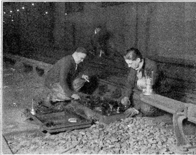
Switch machines are inspected on the first track
