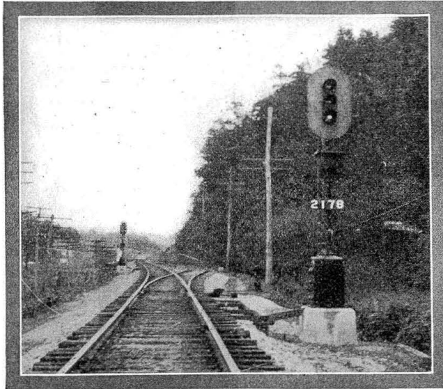
"Head-in" signal at end of siding—Opposing absolute automatic signal in left background
