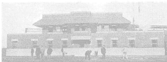
Interlocking tower at Jacksonville, Fla.
