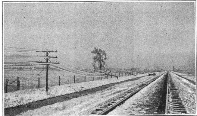
The pole in foreground was guyed four ways and held while all the others in the view went down
