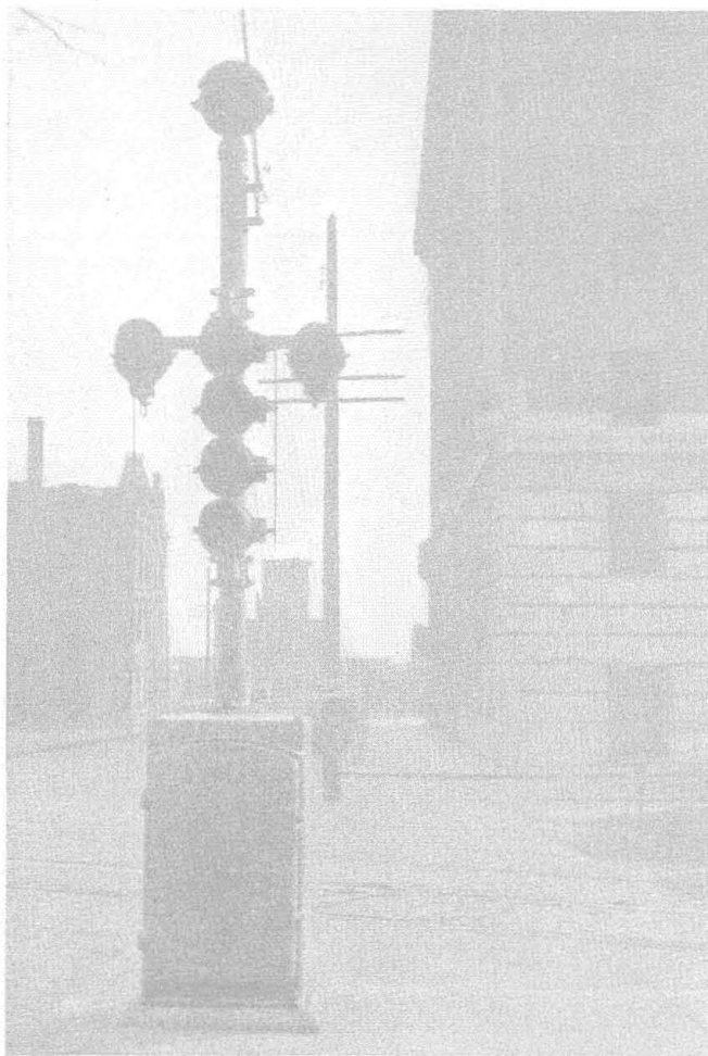
Highway crossing signal at industry tracks of Manufacturer's Railway, St. Louis, Mo.
