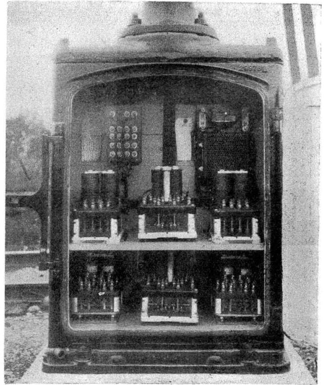
Typical relay case at signal location
