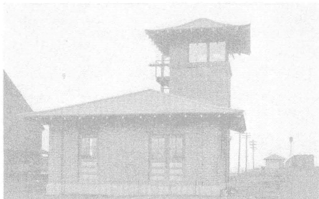
The power house and control tower
