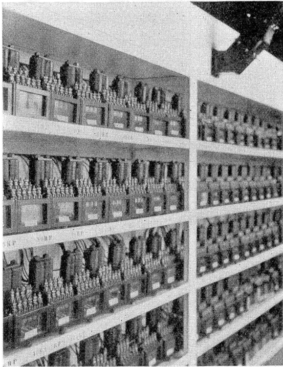
Relay racks—Note Square D conduit leading to machine on floor above
