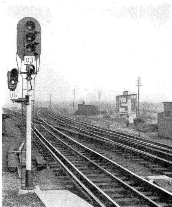
Starting signal U3 and shunting signal U6 at Ruislip
