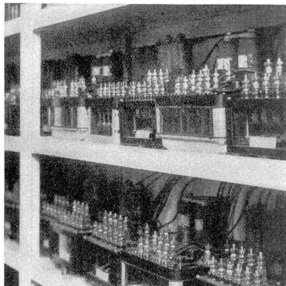
A section of the relay racks
