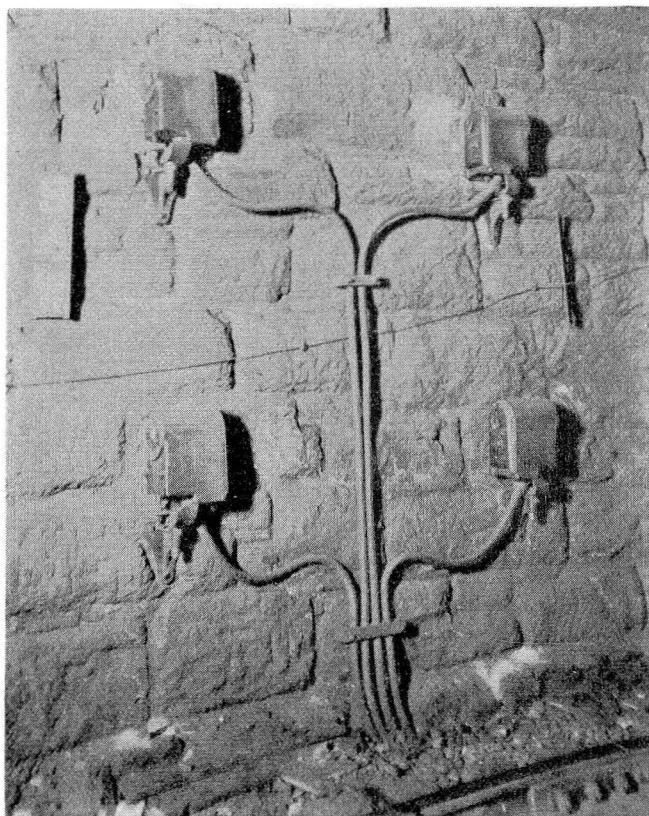
Signal location in tunnel using SA signals for both eastward and westward operation
