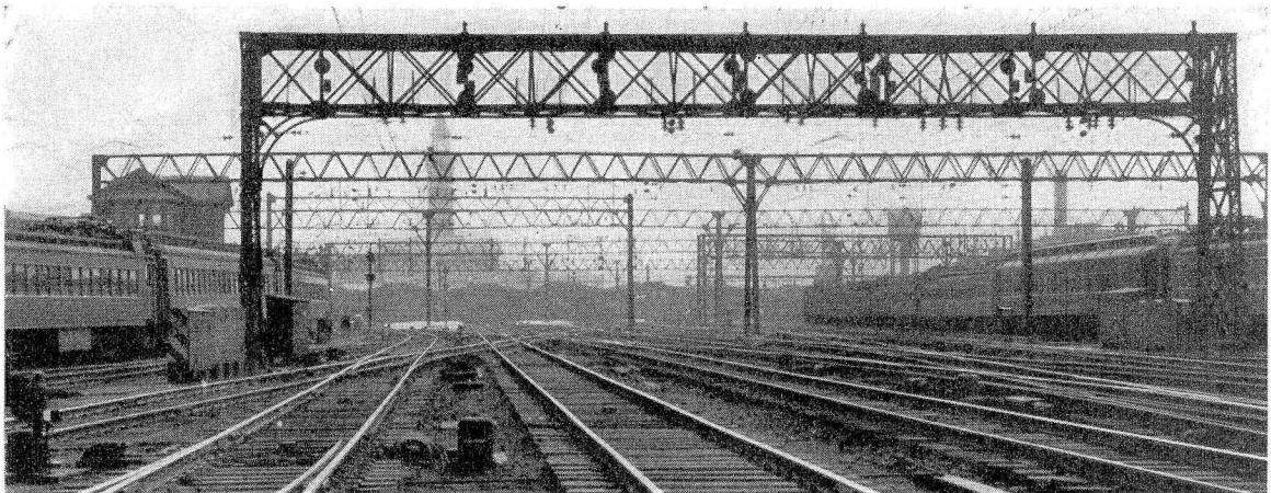
Entrance to Hoboken terminal with combined signal and catenary bridge in foreground—Short-range signals shown here
