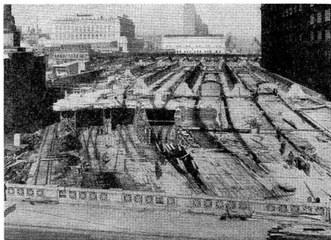
Above—Track level showing false-work covering entire area Right—View looking down on false-work and forms over tracks
