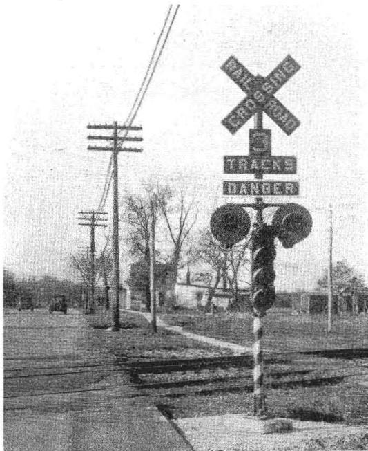
Automatically controlled "STOP" sign and button type crossbuck signs are part of crossing protection
