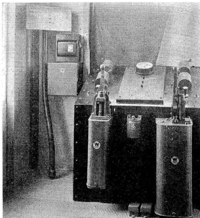
Bridge controller, showing illuminated track and signal diagram at upper left
