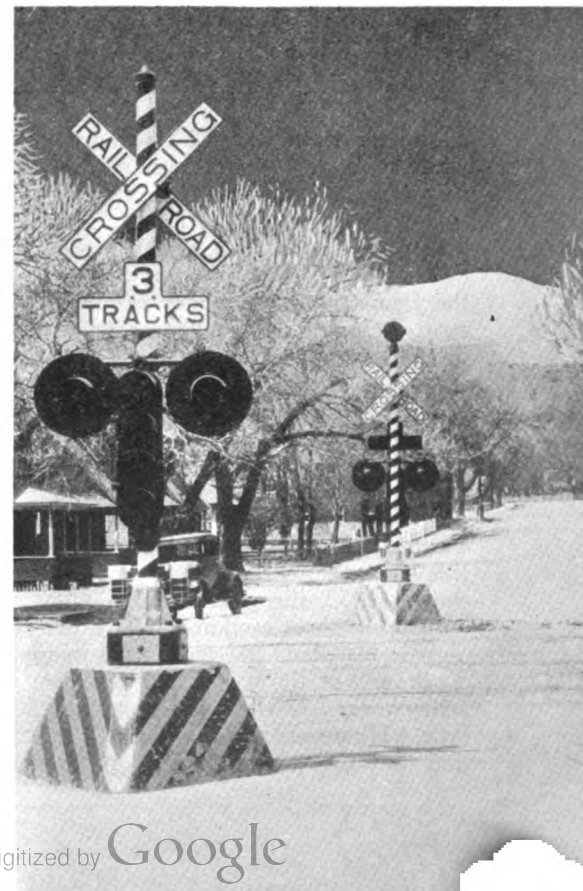
Standard A.R.A. flashing-light crossing signal with automatically controlled STOP sign in service on D. & R. W. in Colorado Springs, Colo., Pike's Peak in background
